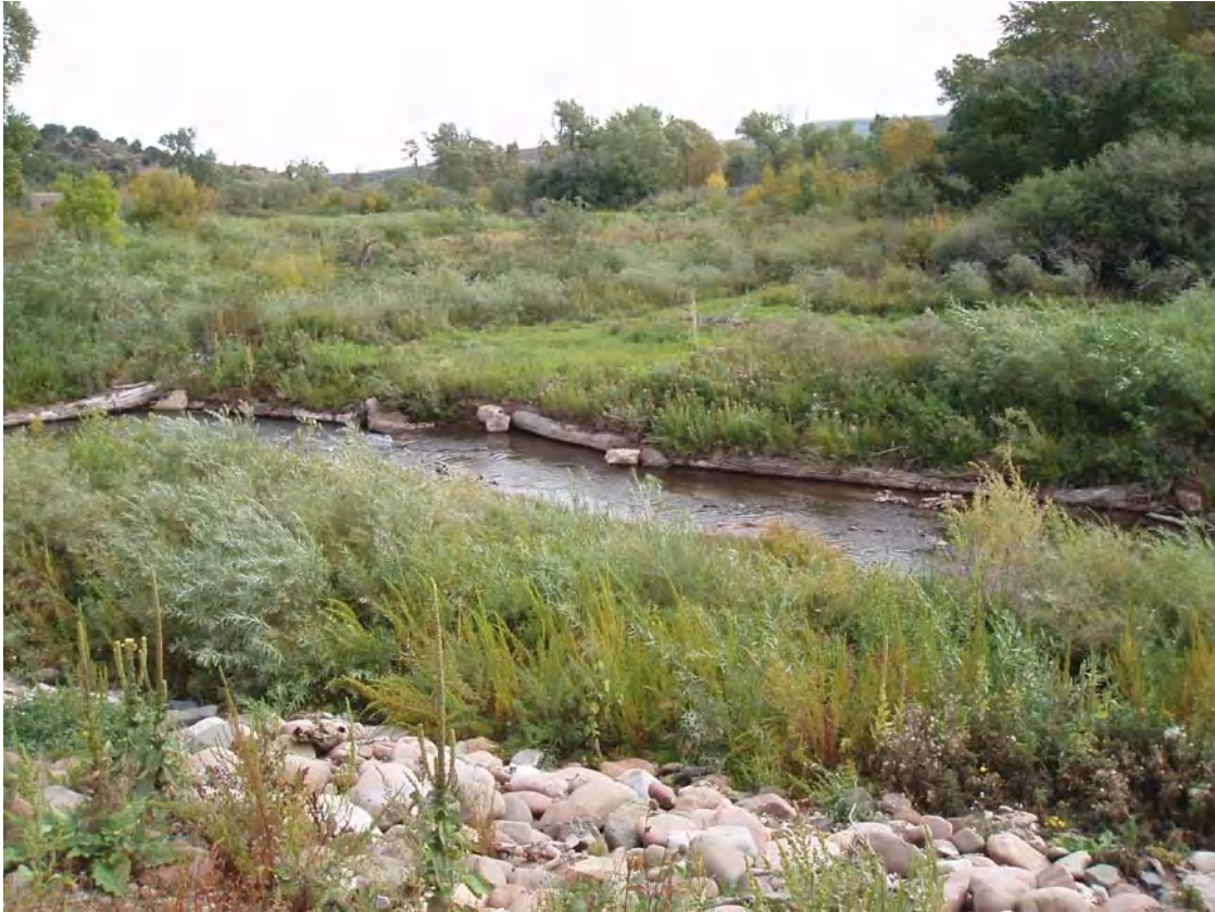
Cottonwood trees used as toe-slope stabilization with riparian benches. Cucharas Creek, Huerfano County, Colorado.
