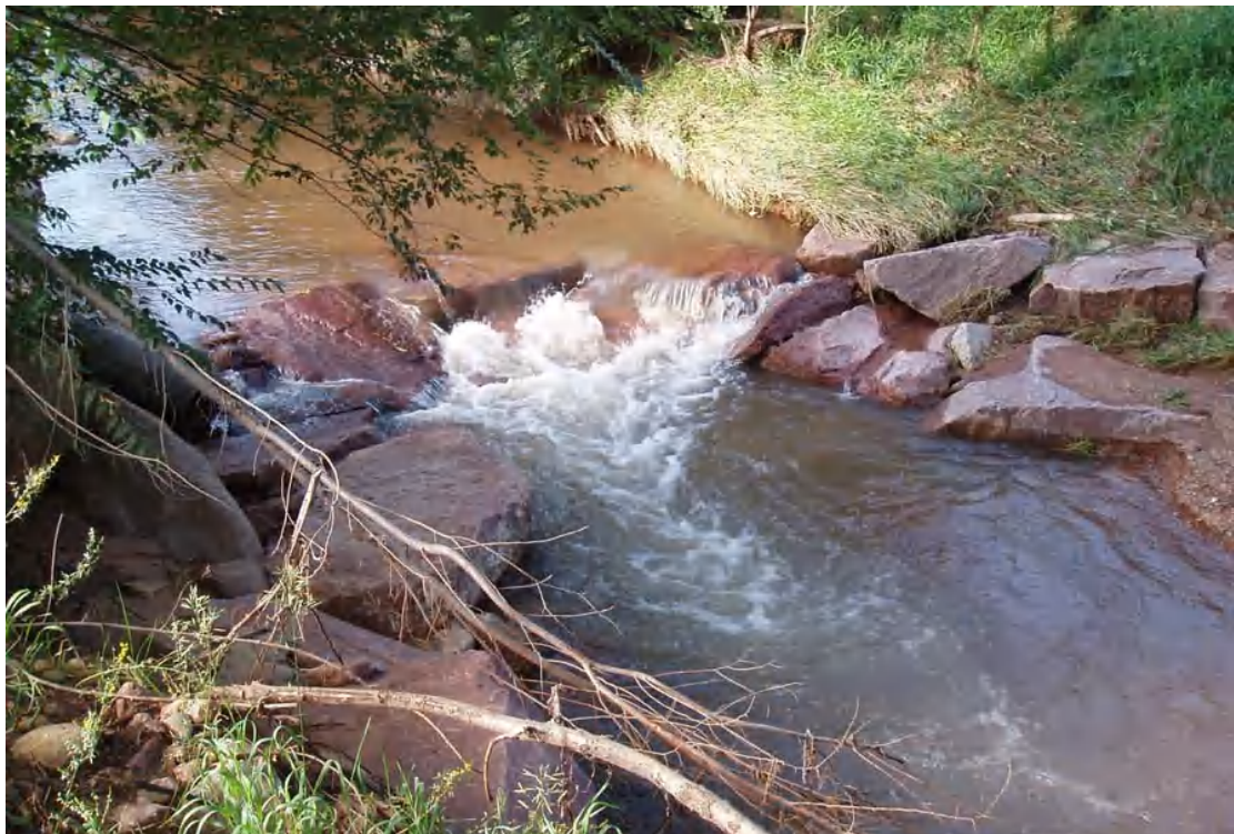
Photo 7: Example of a Boulder Cross Vane Structure - Fountain Creek at 21 st Street.
