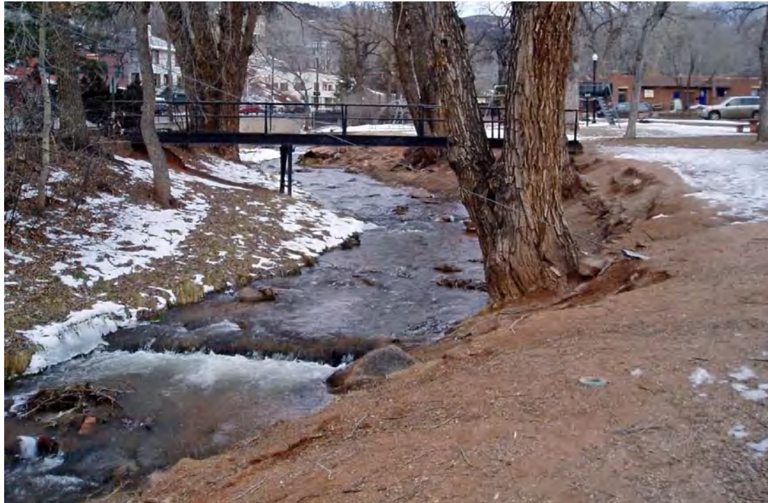
Photo 3: Actively Eroding Stream Banks in the Middle of Reach 11 - Fountain Creek.
