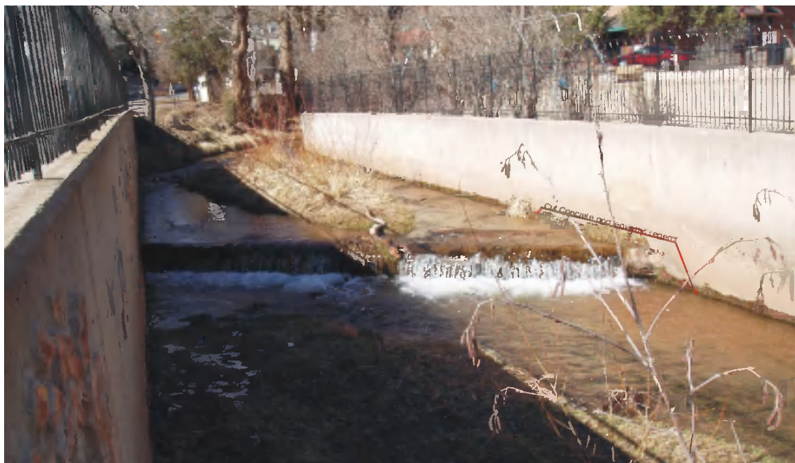
Photo 4: Playground Retaining Wall and Utility Crossing at Log Drop Pool 9
