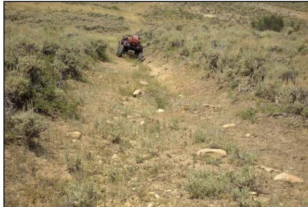
Road erosion due to water channeling in roadway for several years
