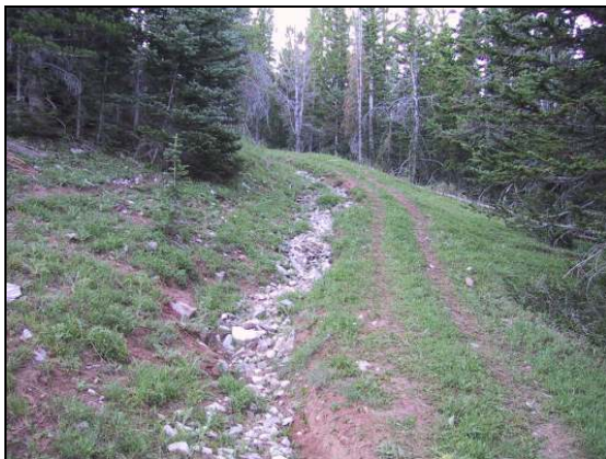
Eroding roadway that needs water diversion to reduce channeling (north side of Mt.)
