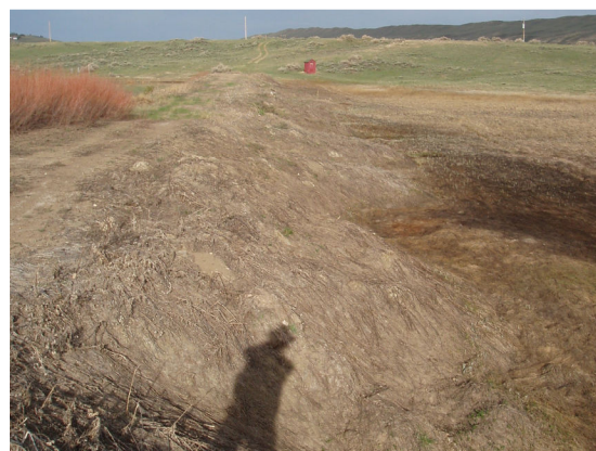
Photo 12: Eroding Downstream side of Dam.
