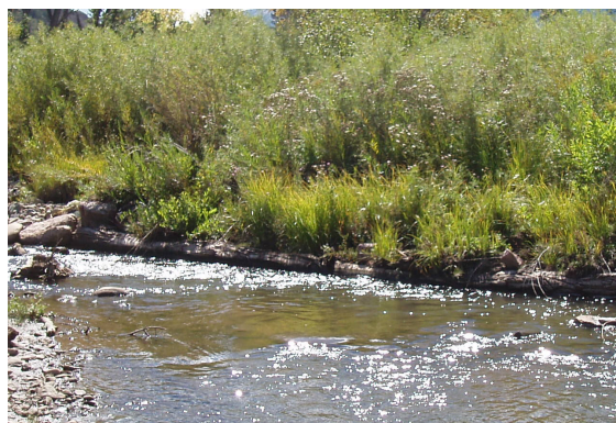
Photo 4: Log toe-slope stabilization of a stream
