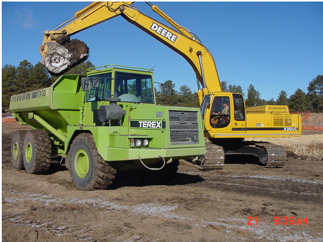
Photo 6: Lake Excavation using a large excavator and 6 wheel articulated dump truck. Manitou Lake, Teller County, CO.
