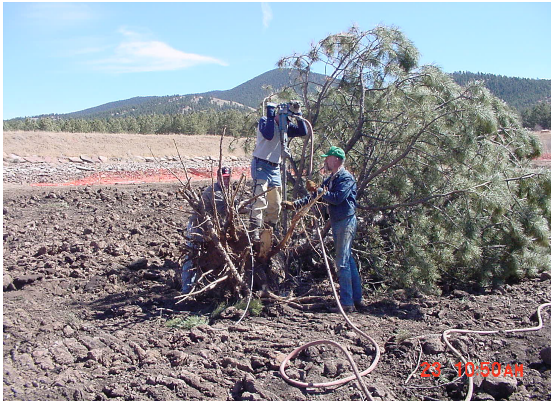
Photo 7: Trout Unlimited volunteers anchor a large pine in the lake bottom using a 90lb pneumatic drill and stainless steel Manta-Ray MR-1 anchors. Manitou Lake, Teller County, CO.
