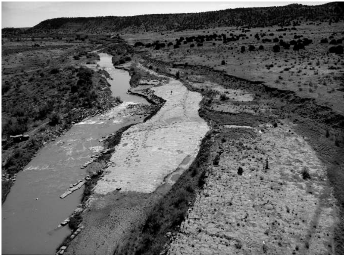
Picketwire Canyonlands, SE Colorado - Rock vanes used to protect dinosaur trackway. These structures were installed in 1998, and survived a 100 year event the following spring. Note the deposition and new willow vegetation taking hold in between the structures. The photo below shows the Project nine years later.
