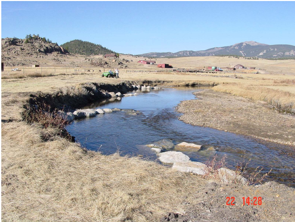
Eagle Rock Ranch - Rock J-Hook Vanes installed to protect stream banks and adjacent road,, 2003.
