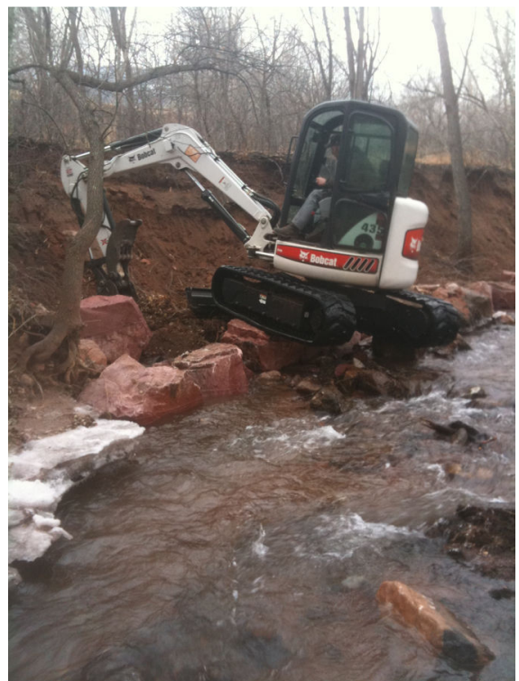
Constructing boulder bank toe in Fields Park.
