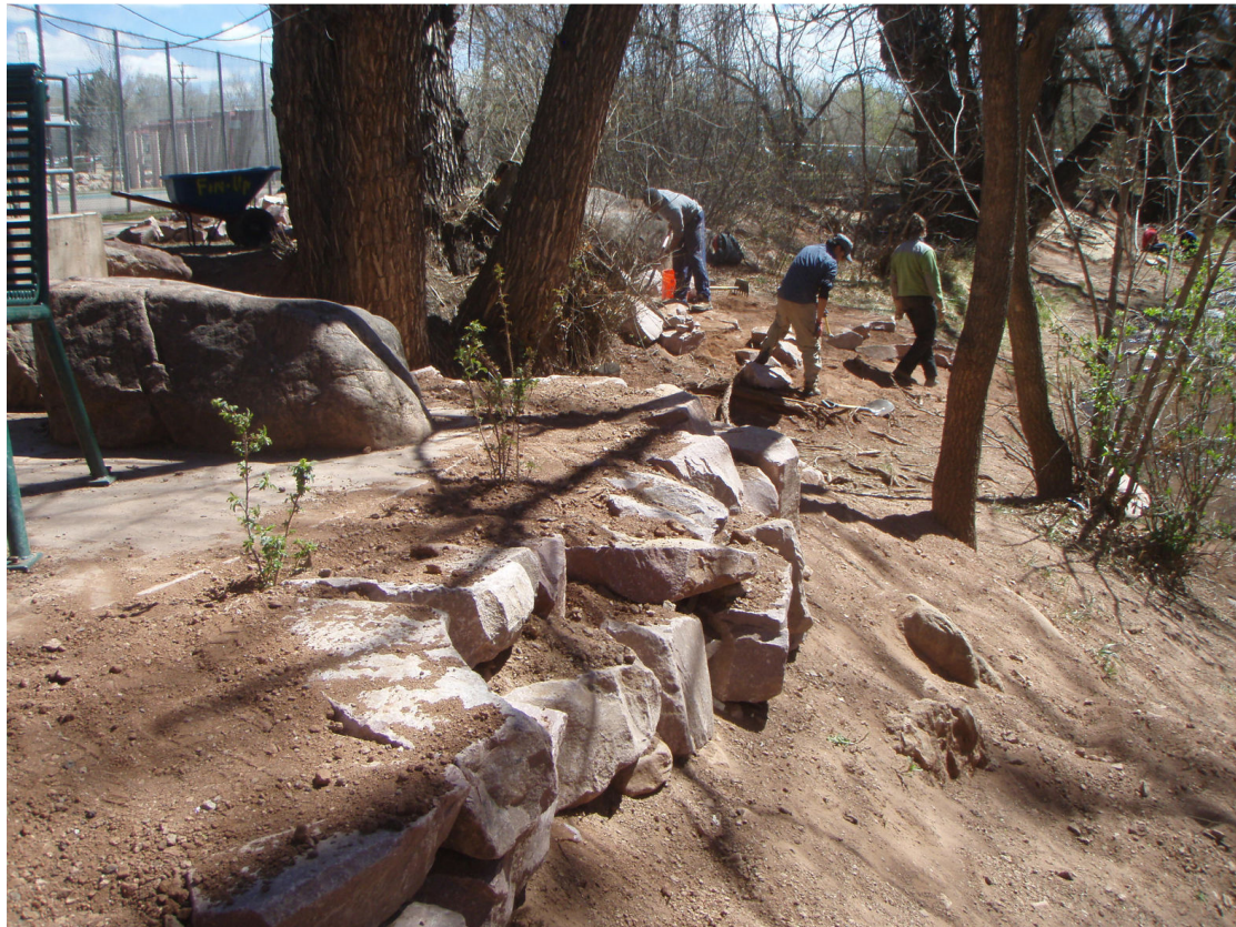
Beginning Stone Wall and Stair Construction in the Lower Part of Fields Park.
