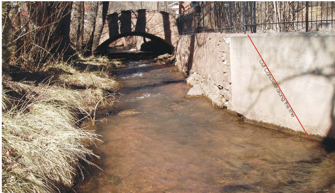
Photo 5: Historic Stone Wall and Interface with Concrete Retaining Wall at Glide 5
