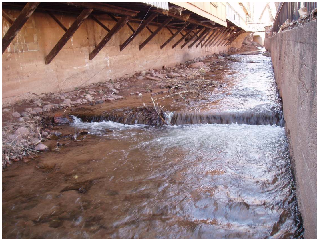
Photo 6: Concrete Retaining Wall Channel Downstream of the Stone Bridge - XS#1.
