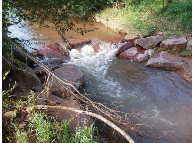
Photo 7: Example of a cross vane structure constructed to stabilize the vertical profile of the river channel. Fountain Creek below the 21 st Street Bridge. Colorado Springs, El Paso County, CO
