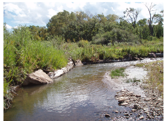
Photo 9: The same bank on Cucharas Creek one year after toe-slope logs were installed in Oct. 2005
