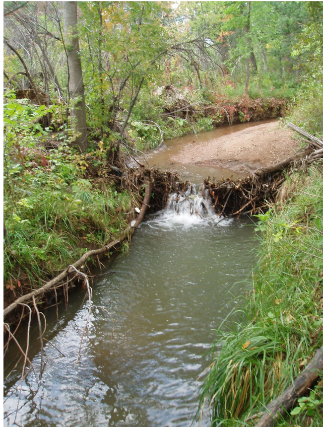
Photo 3: Plunge Pool 12 on Reach 2 - Bear Creek. Note sediment in storage in the channel upstream of the pool.
