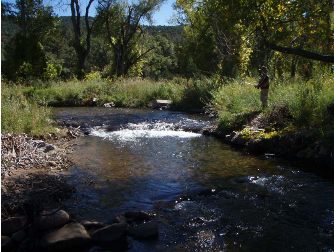
Double Log Cross Vane with Restored Stream Bank Upstream - Beaver Creek Wildlife Area, CO.
