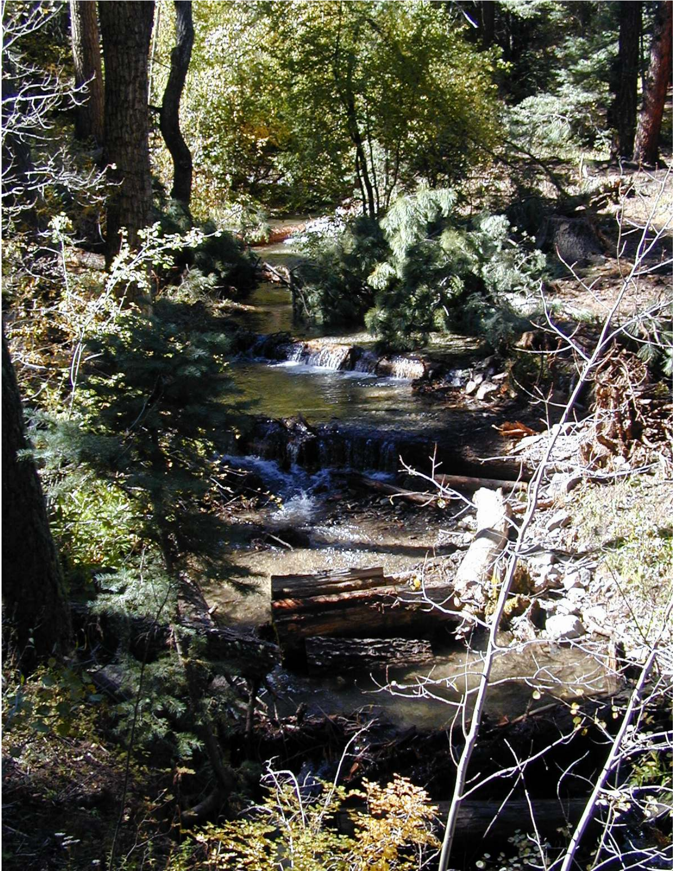
Freshly Constructed Step-Pool System - South Prong of Hayden Creek, Freemont County, CO.
