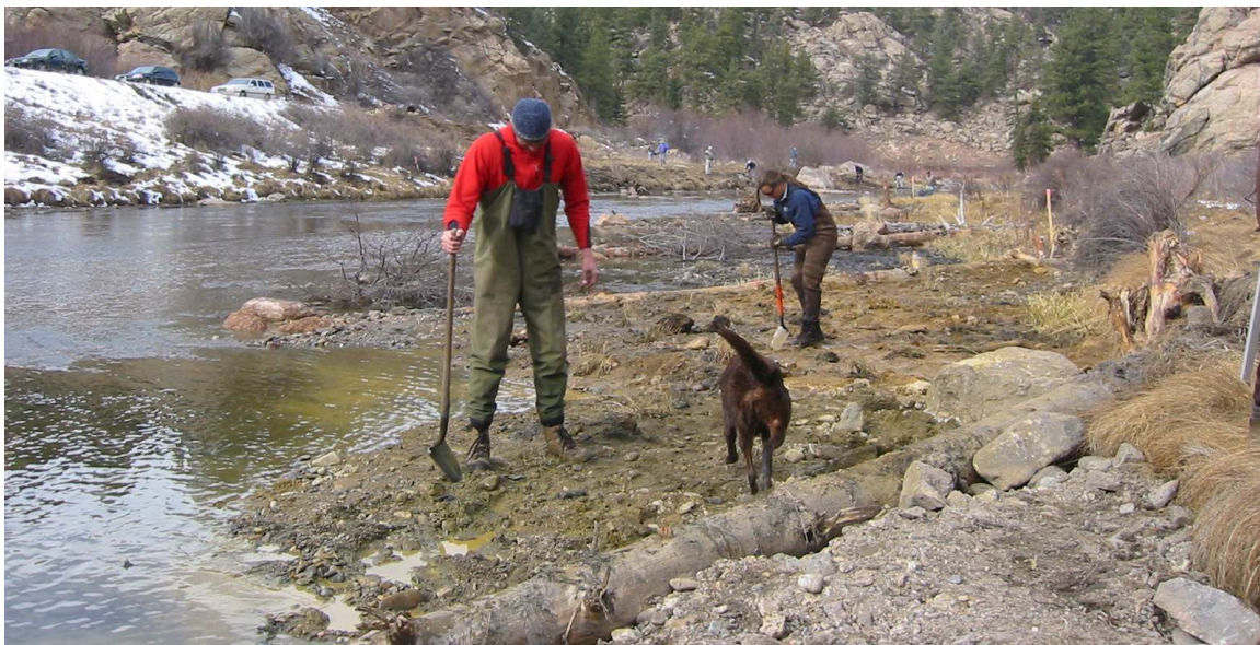
Large Wood installed low in the channel to reduce Width/Depth Ratios - South Platte River, Eleven-mile Canyon, IFIM Middle Station. 2004 " Trees for Trout " Demonstration Project
