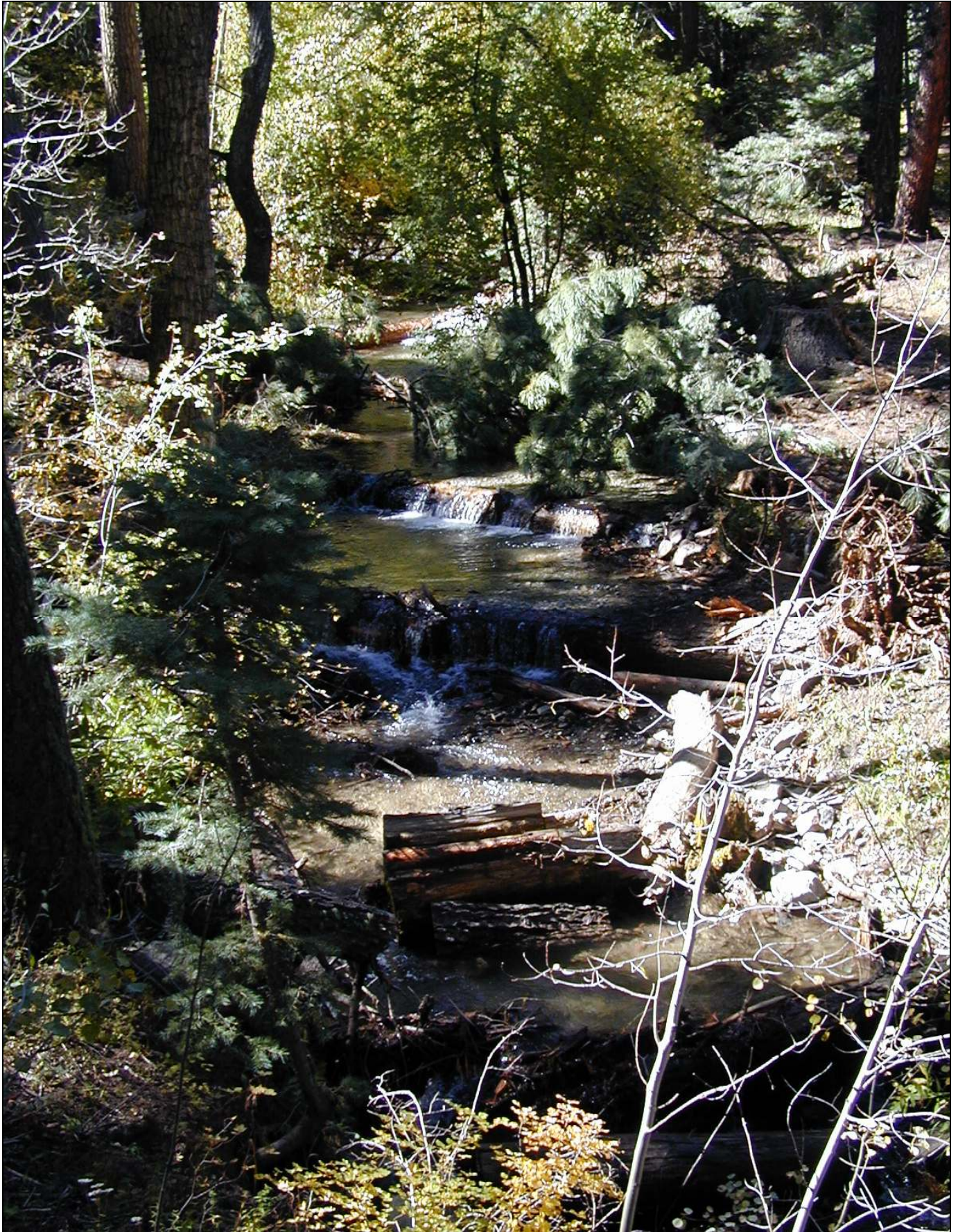
Newly Constructed Step-Pool System in a Greenback Cutthroat Stream - S. Prong of Hayden Creek, Freemont County, CO.
