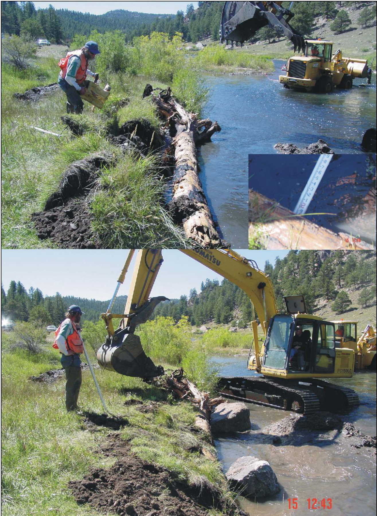
Constructing a LUNKER Stream Bank and Riparian Bench Structure - Elevenmile Canyon Trees for Trout Centennial Project.
