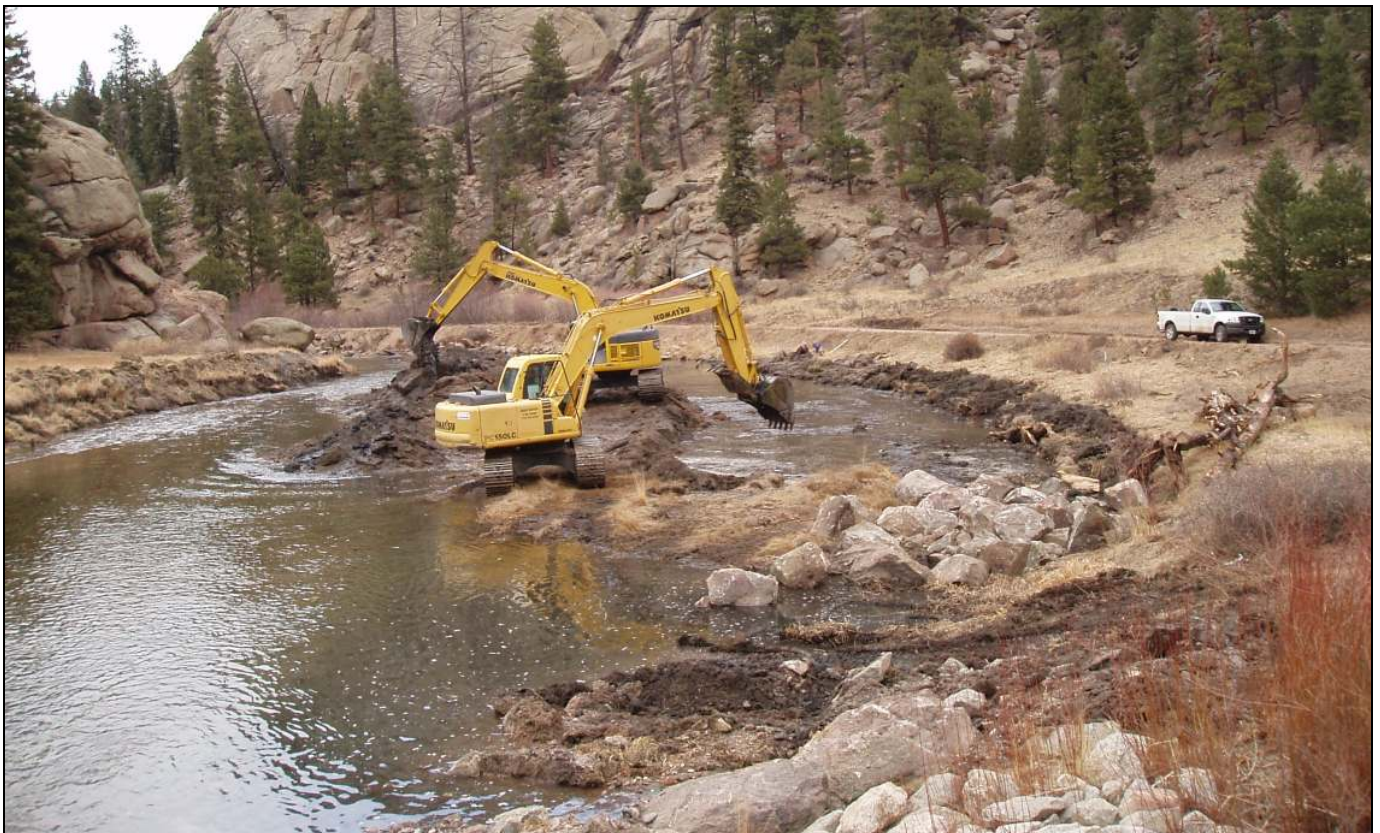
Removing the Mid-Channel Island - Elevenmile Picnic Ground Channel Reconfiguration Project - South Platte River.
