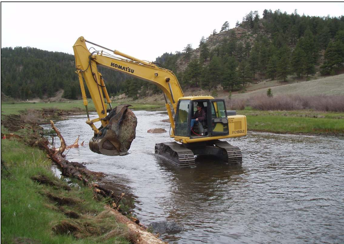
Installing Bank Full Bench & Log Toe Slope Structure - South Platte River, Camp Alexander, Park County, CO
