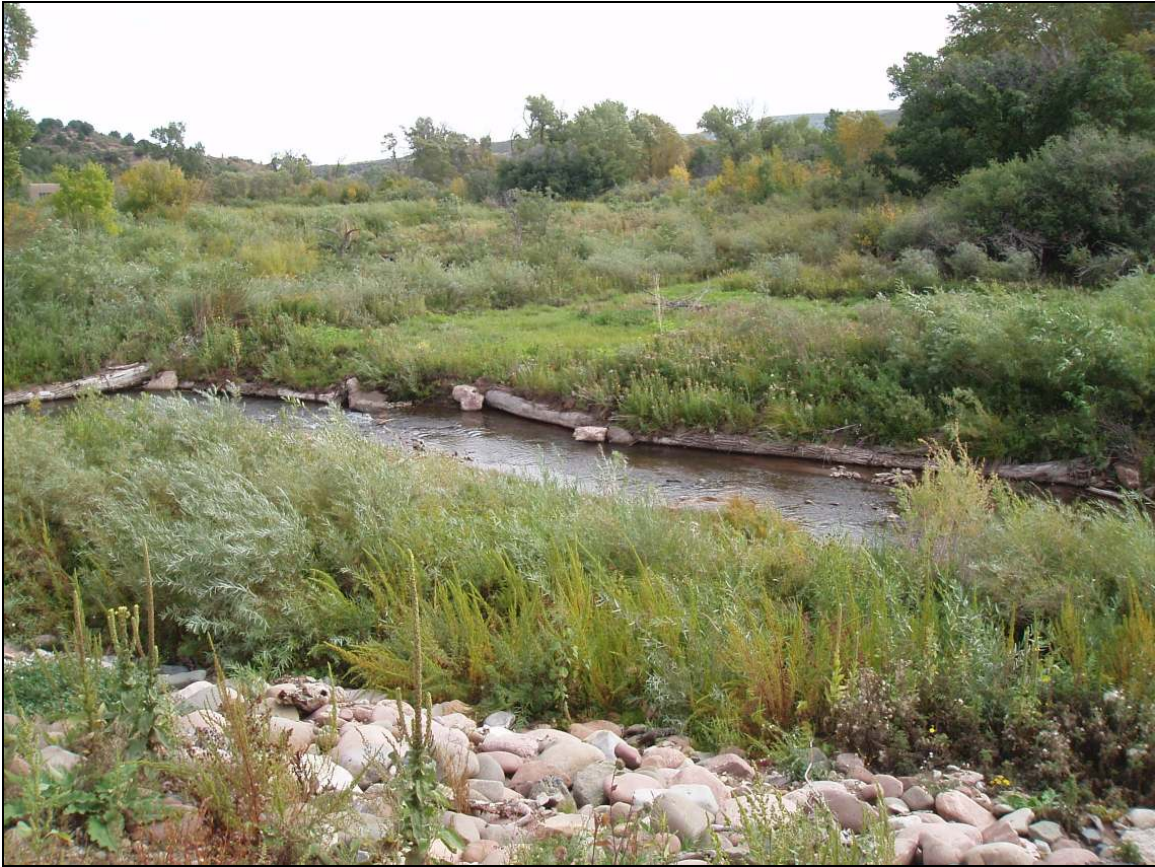
Riparian Bench / Log Toe Slope Structures, one year after construction - Cucharas River, Huerfano County, CO.
