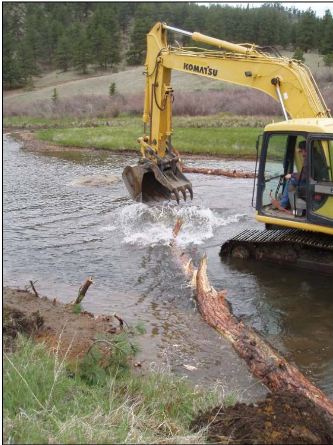
Installing a Log Vane - Camp Alexander, Elevenmile Canyon. Elevenmile Picnic Ground Channel Reconfiguration Project.
