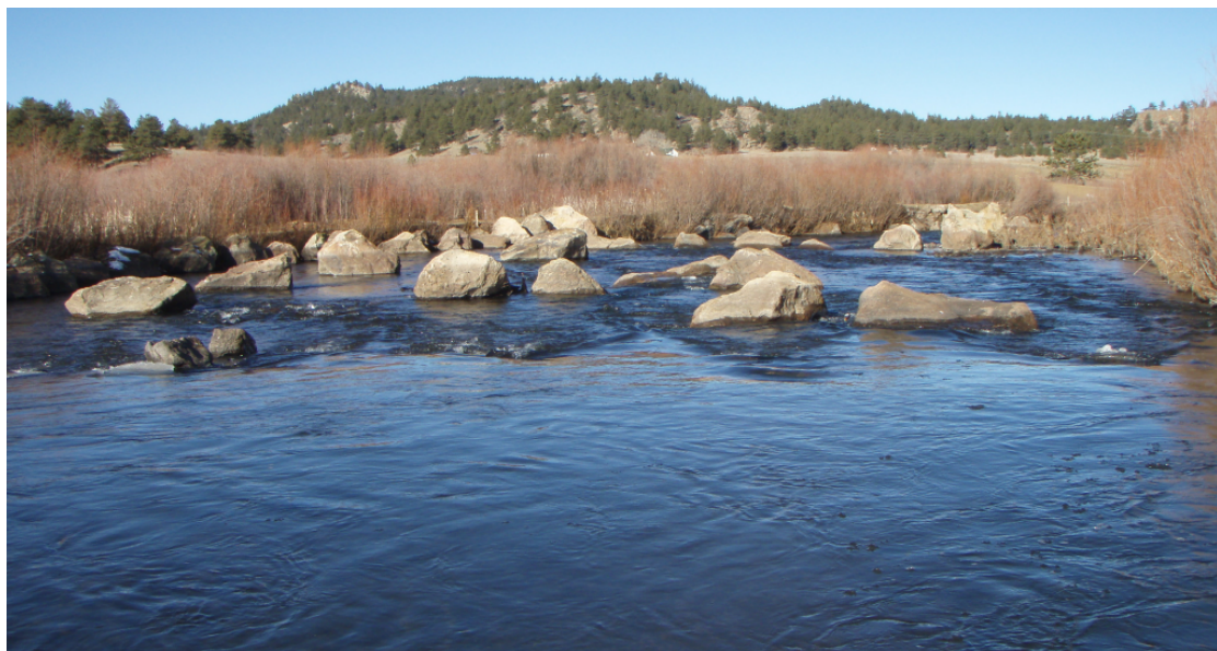
Photo 2: Boulder Clusters in Structure #9 with Bank Structure #8 in background.
