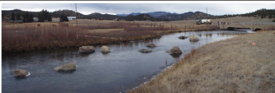
Photo 1: Typical Random Boulder Cluster Structure in Reach 1, South Platte River.
