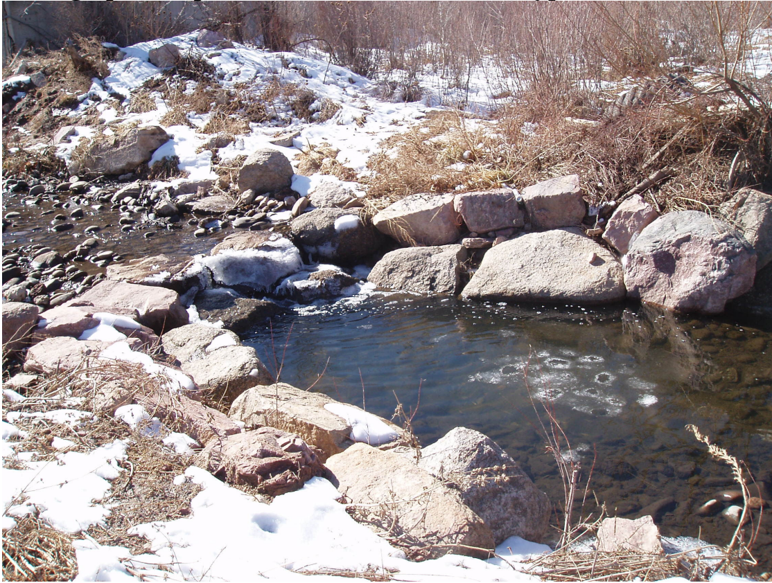
Cross Vane Structure on Cheyenne Creek below I-25 Overpass. Colorado Springs, El Paso County, Colorado
