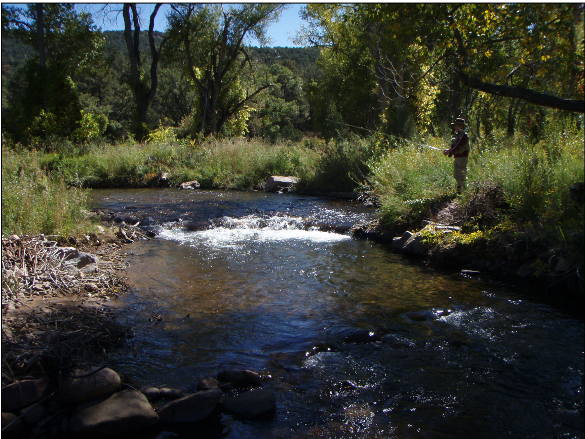
Double Log /Boulder Cross Vane with Restored Stream Bank Upstream - Beaver Creek Wildlife Area, CO.
