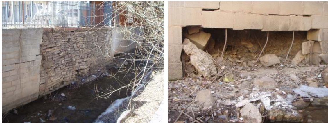
Photos 16 & 17: Failing retaining walls at the Pikes Peak Inn, within Sub Reach 7c.
