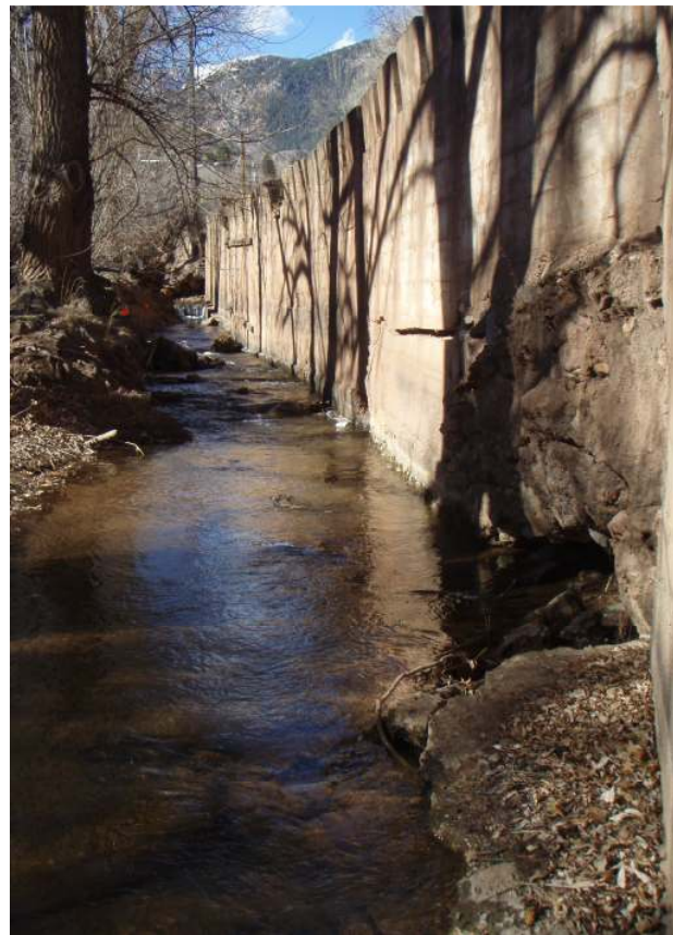
Photo 7: Unusual combination cover formed by failing concrete retaining wall footings - Lover's Lane retaining wall - Reach 7.
