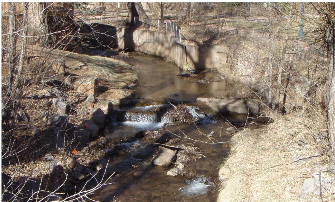
Photo 3: Concrete block drop structure - Mansions Park behind City Hall.
