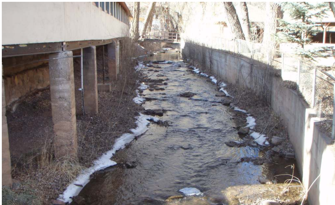
Photo 14: Fountain Creek adjacent to City Hall, looking upstream. The eroding foundation can be seen on the left side of the photograph.
