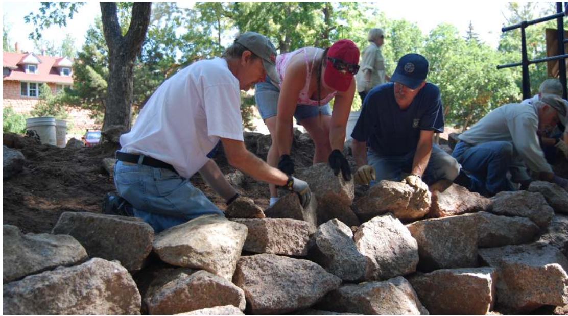
Photo 12: Volunteers constructing terrace walls for revegetation of stream banks. Similar techniques will be used in Sub Reach 7a to stabilize stream banks.
