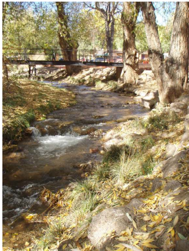
Photo 9: Restored stream bank and cross—vane. Soda Springs Park Reach 11 on Fountain Creek.
