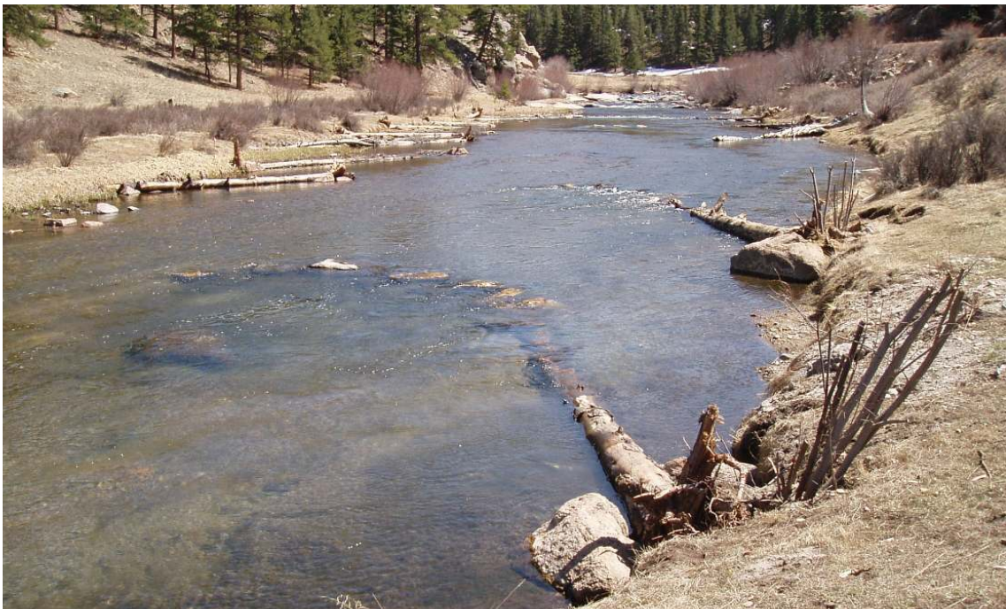
Photo 23: Large wood / boulder J-Hook Vanes - South Platte River, Elevenmile Canyon, IFIM Springer Gulch Middle Station. 2004 "Trees for Trout" Demonstration Project
