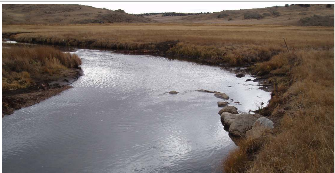
Photo 28: Example of a boulder J-Hook Vane. Tarryall River – Eagle Rock Ranch, Park County, CO
