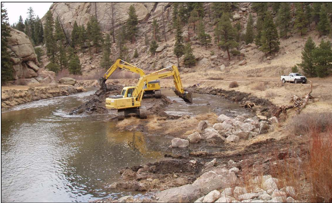
Photo 25: Island removal and river narrowing project. S. Platte River - Elevenmile Canyon PG - 2006
