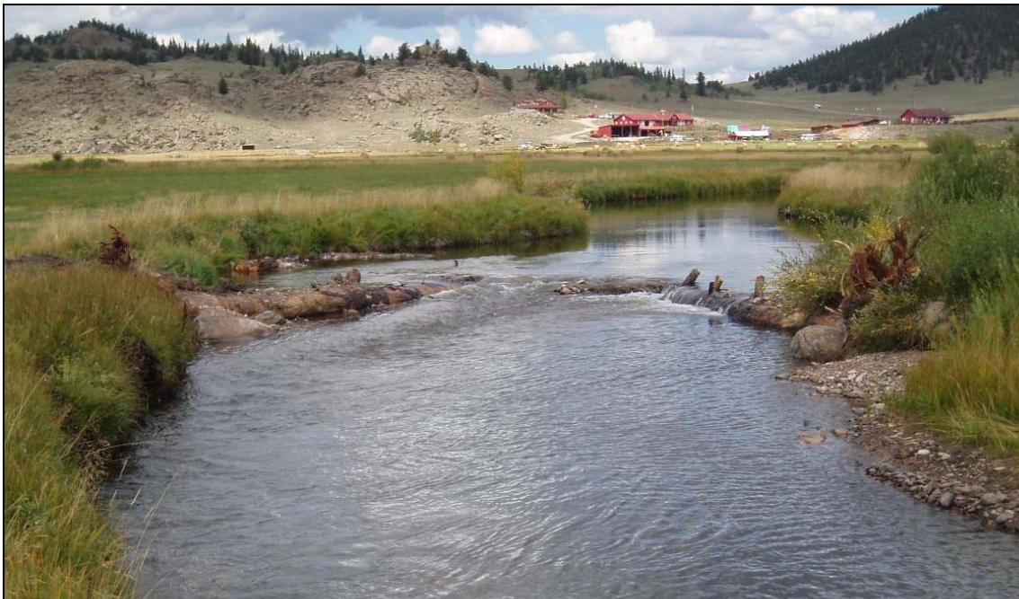
Photo 23: Double Log /Boulder Cross-vane Structure - Eagle Rock Ranch, Tarryall River, Park Co., CO
