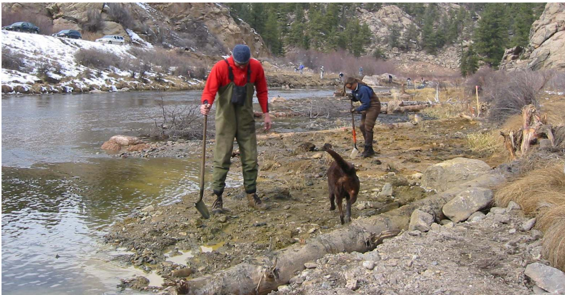
Photo 18: Large wood installed low in the channel to reduce width/depth ratio - South Platte River, Elevenmile Canyon, IFIM Springer Gulch Middle Station. 2004 " Trees for Trout " Demonstration Project
