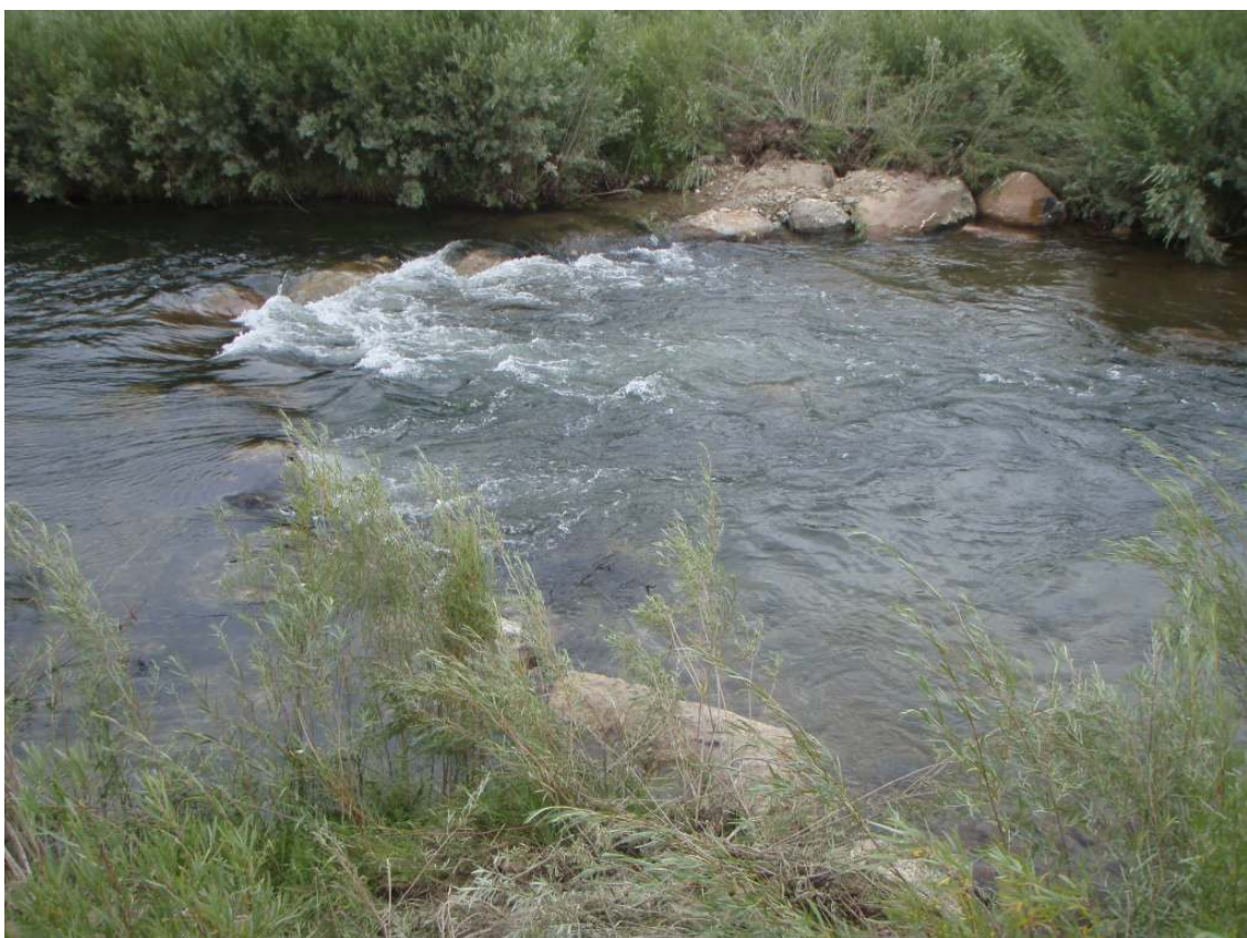
Photo 21: Full Channel Boulder Cross-vane. South Platte River at Lake George, CO.
