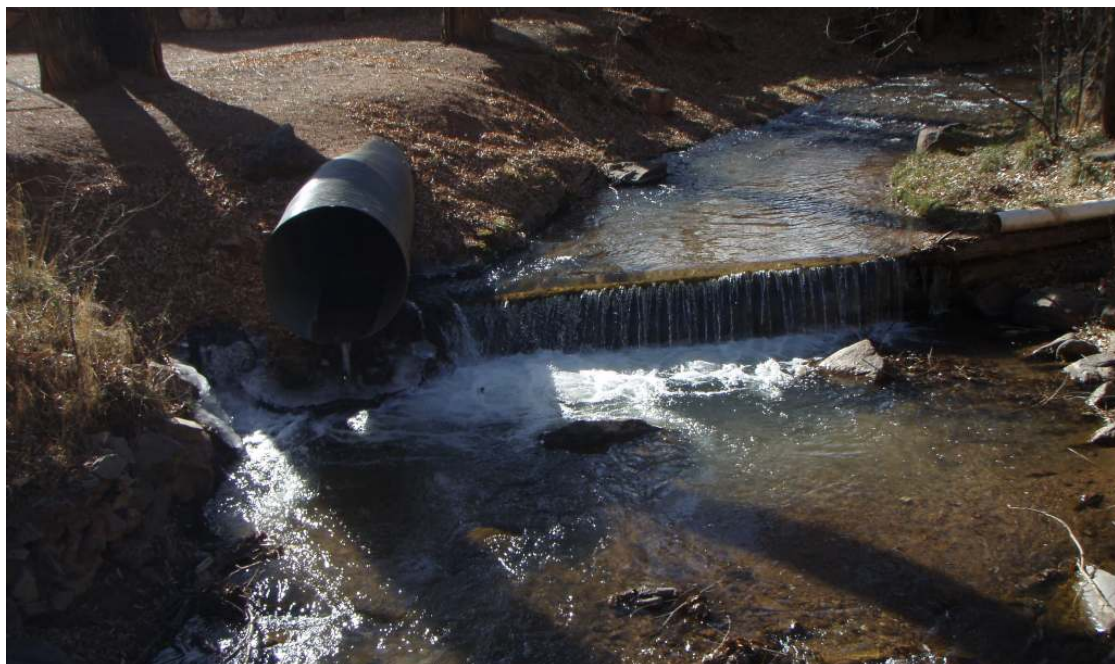
Photo 2: Diversion structure and potential fish barrier on Reach 4 - Shryver Park.
